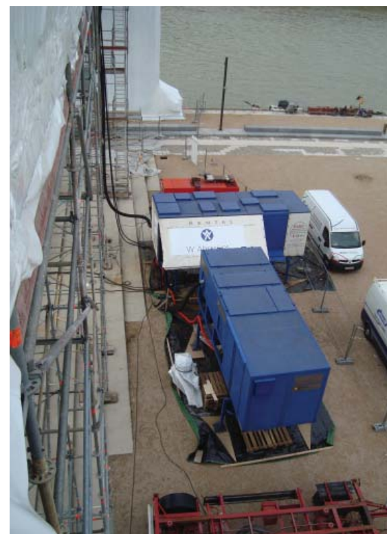
PHENICS mobile equipments on work-site
