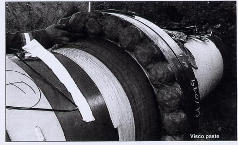
The material is made of amorphous a-polar polyolefins with no reactive groups and free radicals. It has an extremely low permeability for water and is impermeable for moisture under ambient conditions. Due to the amorphous structure, the coating will wet the surface of the substrate up to a physical molecular level.
