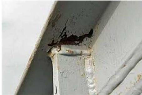
Typical example of detrimental effects of soluble salts under a coating system (surface corrosion). Osmotic blistering (*left*); loss of adhesion due to underfilm corrosion (*right*).
